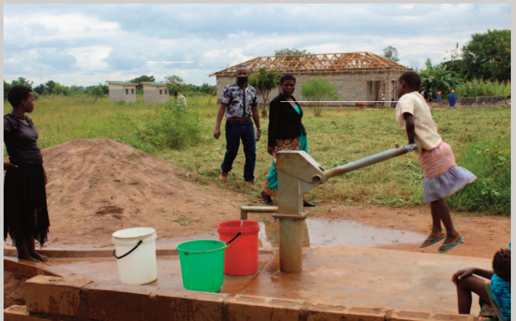
Borehole at the construction site
