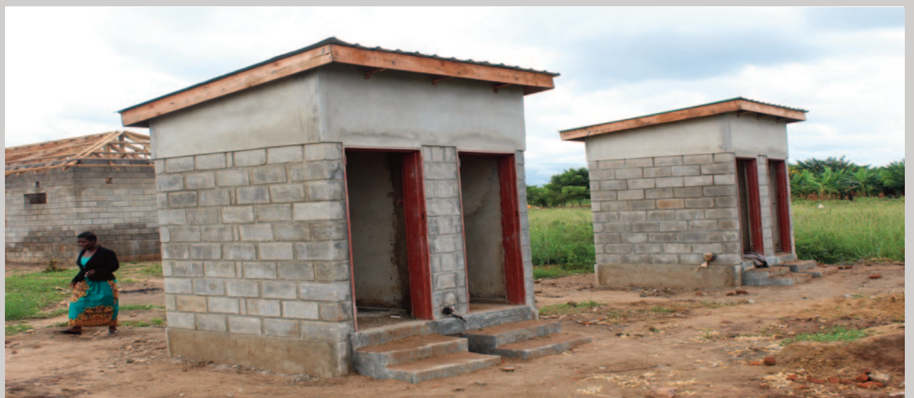
Community centre toilets
