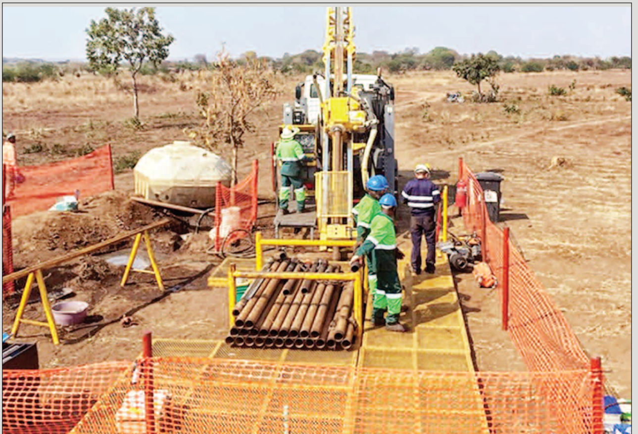
Drilling work at the Malingunde site
