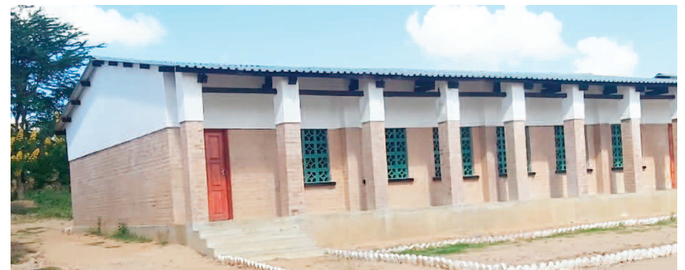
School block constructed at Chigumba Primary School
