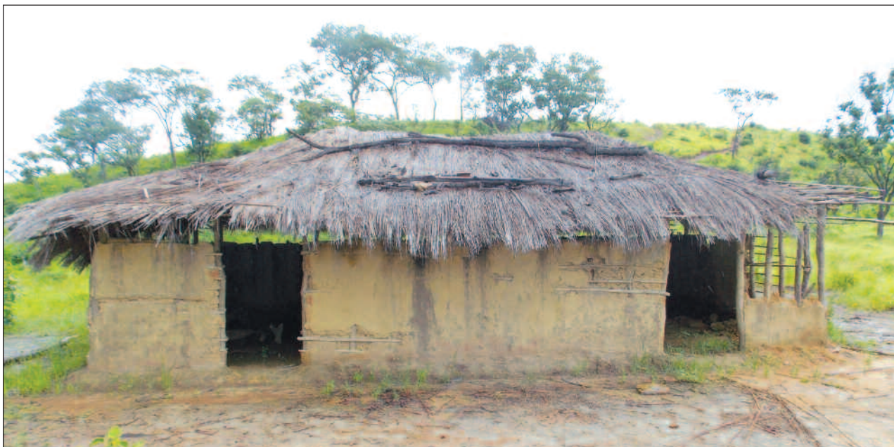
Self-help initiative: A junior primary school that the Gondwe Clan constructed for their children
