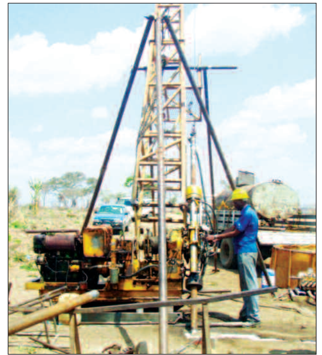
Drilling works at Kanyika
