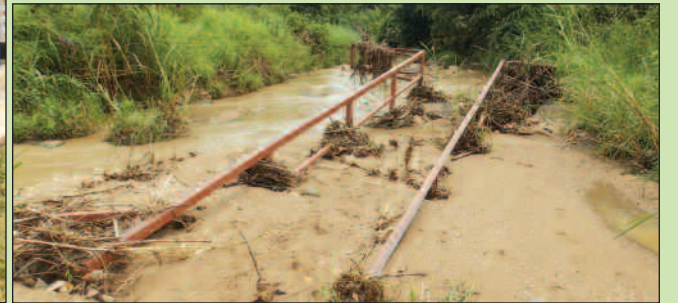
Washed-away bridges at Kayelekera area
