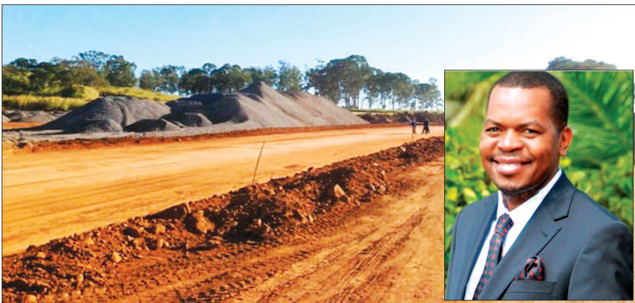
Road construction works underway and inset is Hiwa, Roads Authority CEO
