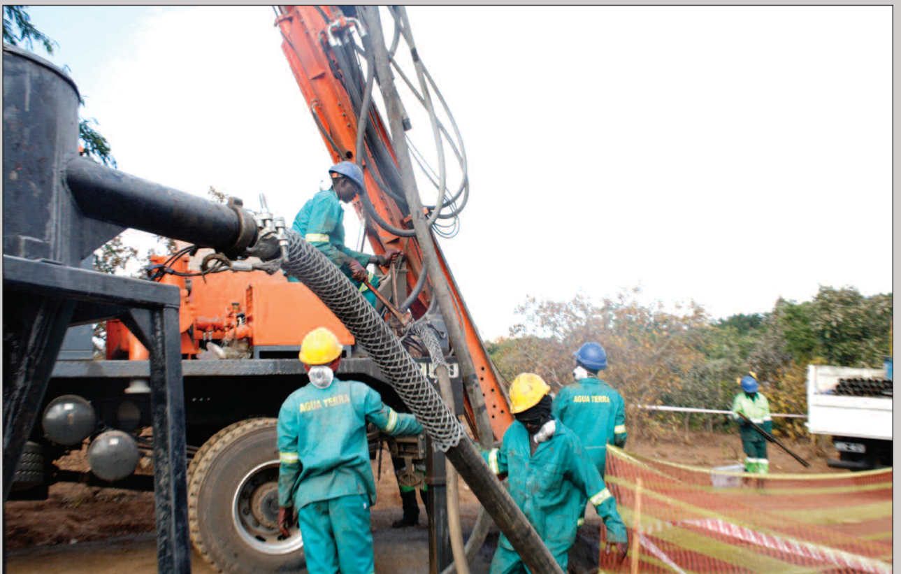
RC drilling at Duwi Main
