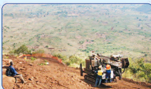
Moving Drill Rig to Drill Pad
