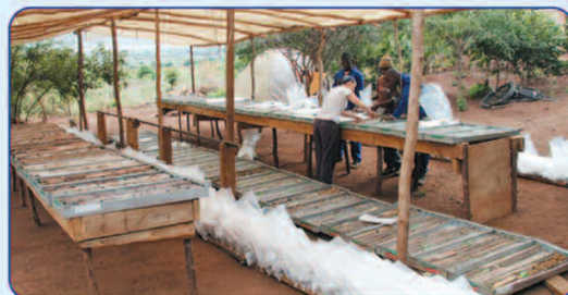
Sampling work underway
