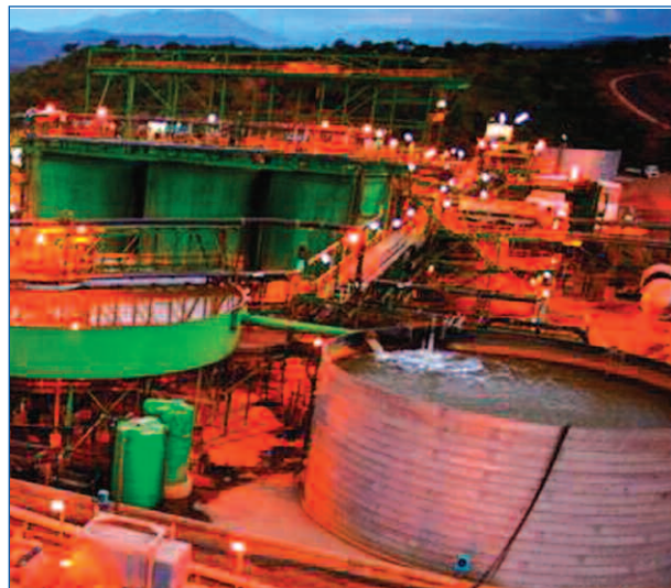
Standard Bank financed Kayelekera Uranium Mine
