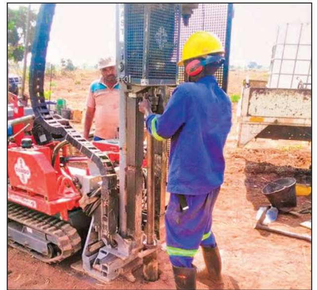
Drilling in progress at Kasiya
