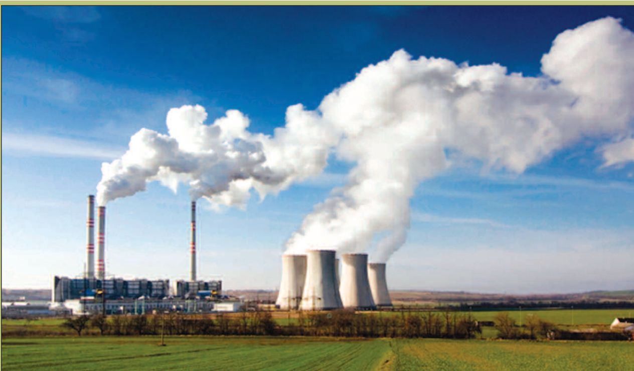
Operational coal power plant: Will Malawi have similar infrastructure?
