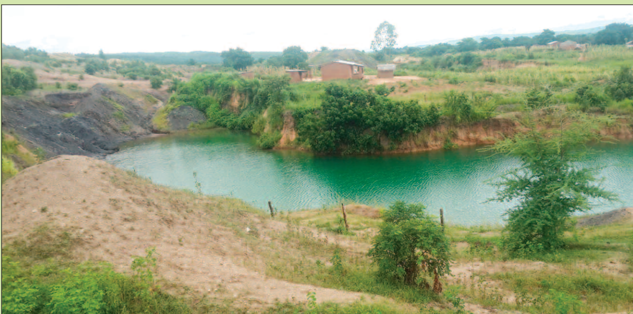
Community facing danger of drowning in several of these gullies that are filled with water
