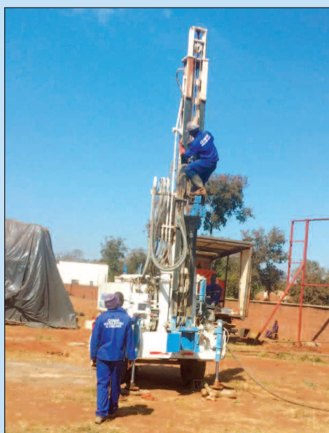
Experts setting up a water drilling machine
