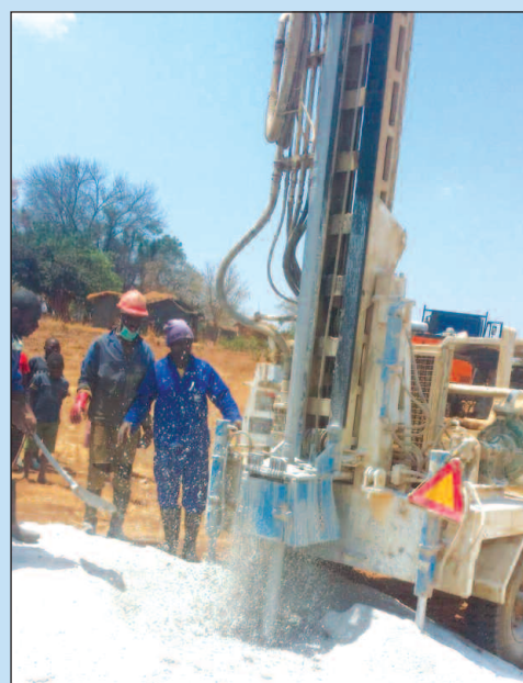
Water drilling works in progress
