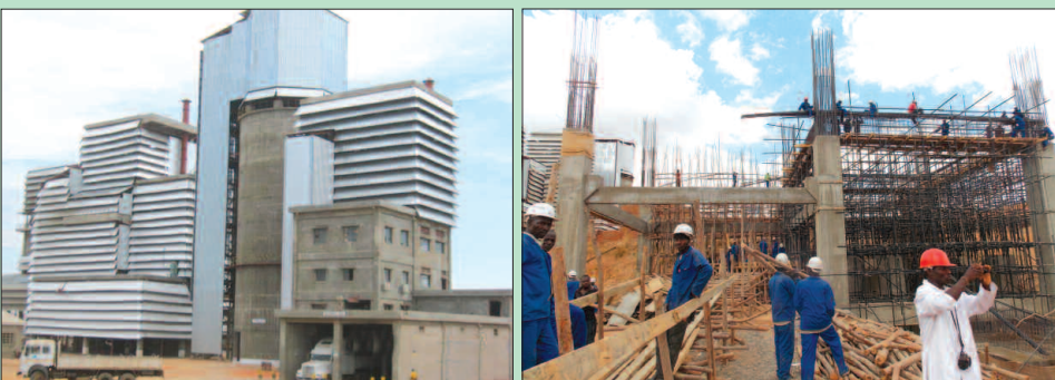
New cement manufacturing plant
