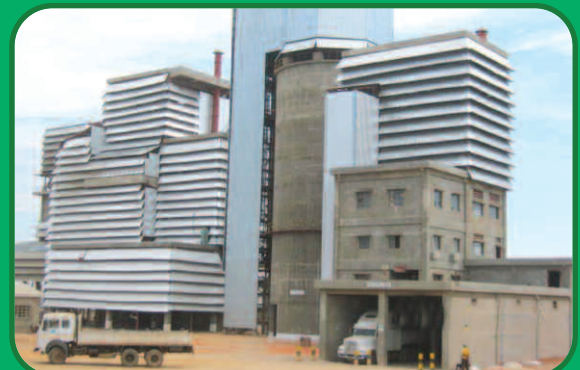
Part of the Shayona Cement Corporation new plant in rural Kasungu
