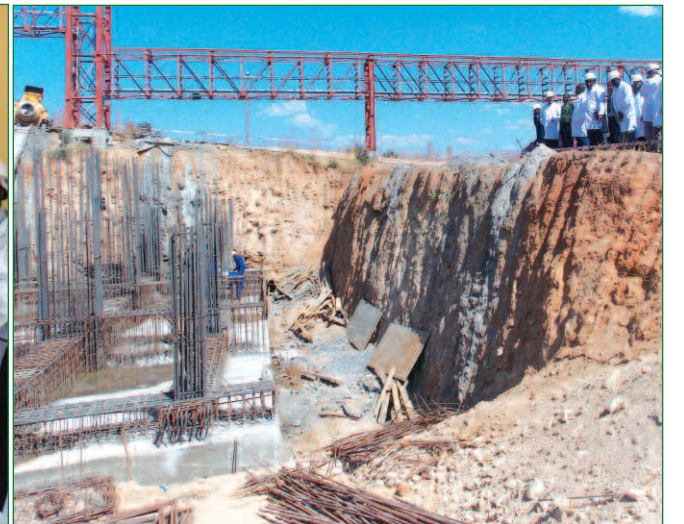
New development works at the factory
