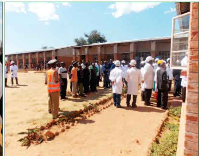
Social responsibility: School blocks that Shayona constructed
