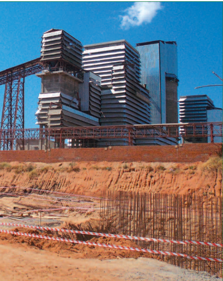
Plant in progress
