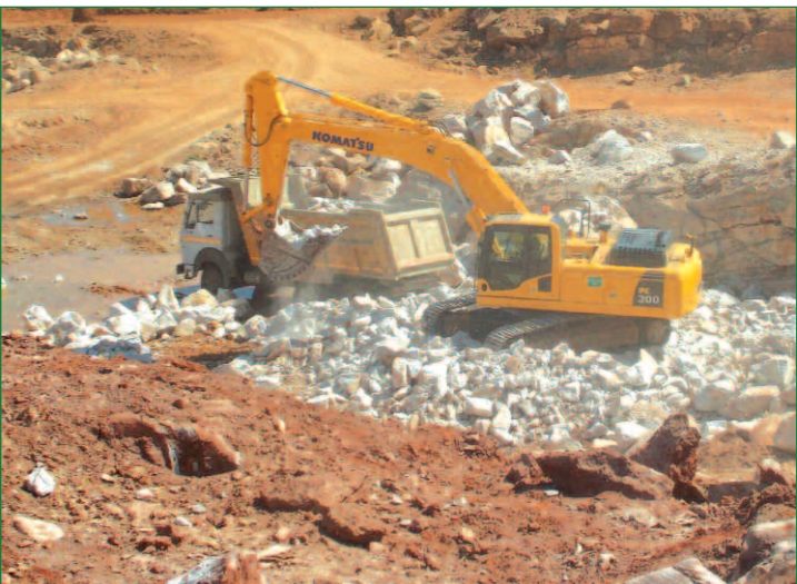
Work at the mine on course
