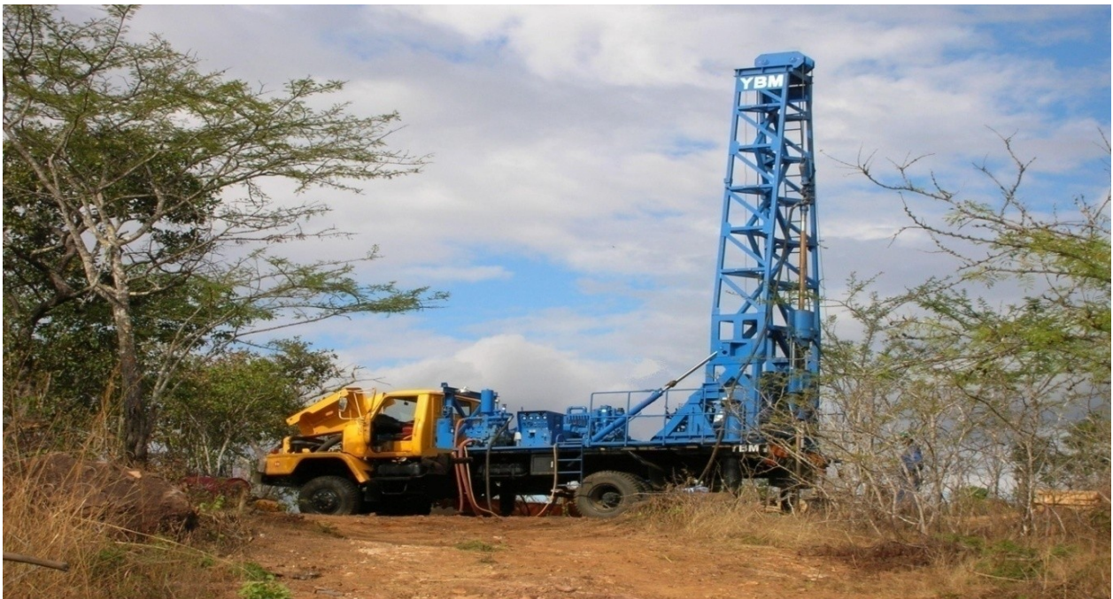
Exploratory drilling in progress
